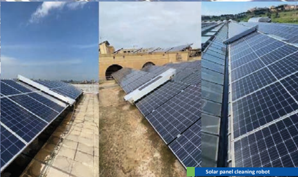
Solar panel cleaning robot
